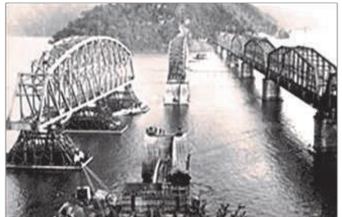
Construction of second bridge
