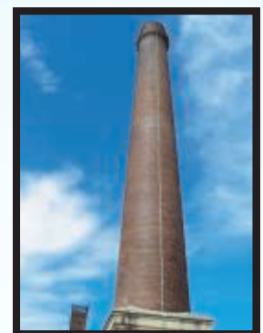
We had to guess how many bricks were laid in this chimney.
