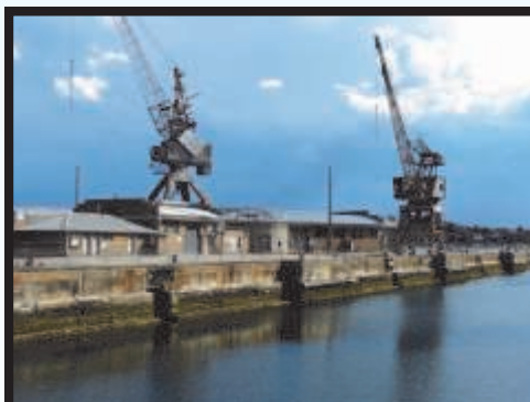
There are several old cranes still installed on the Island
